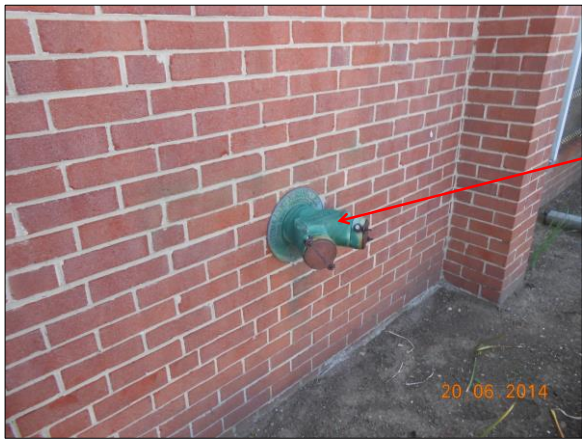
Photograph 47 4" Piping (Fire Department Connection), Exterior, Lead Paint
