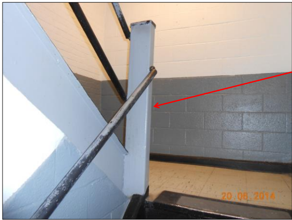
Photograph 40 Railing Post, Room 23, Lead Paint
