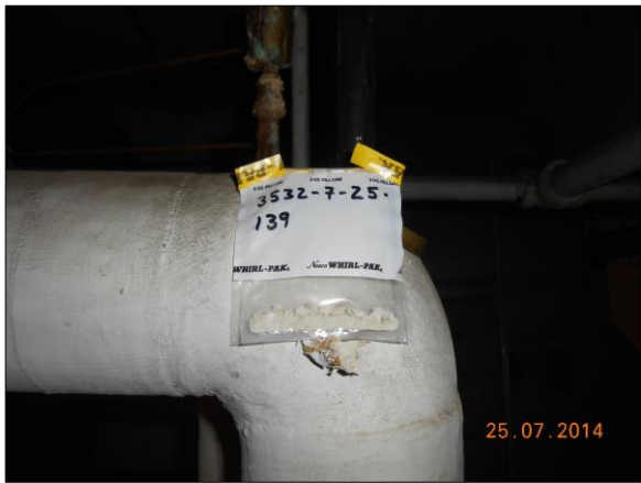
Photograph 33 4" Fitting (TSI5), Room 134, Positive 2% Amosite, Trace Chrysotile
