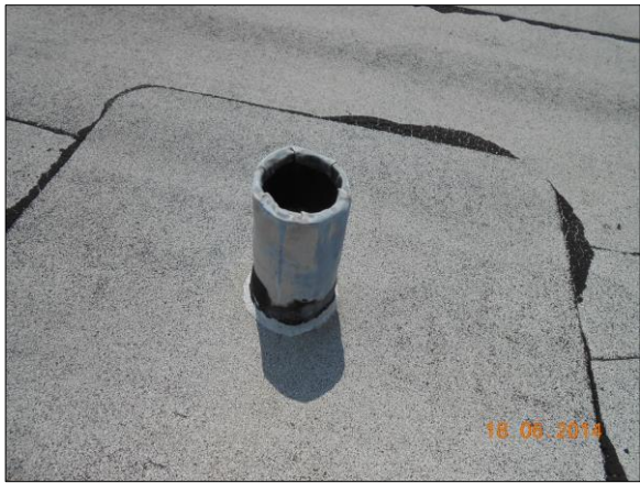
Photograph 68 Lead Vent Pipe, Exterior Roof, Miscellaneous Material
