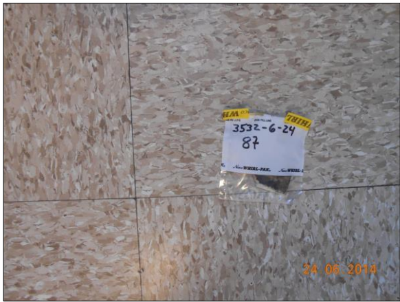
Photograph 22 Floor Tile (FT5), Room 47, Positive 2% Chrysotile Floor Tile Mastic (FT5), Room 47, Positive 4% Chrysotile
