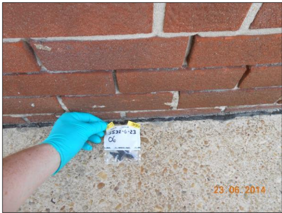
Photograph 13 Expansion Joint (OM14), Exterior of SUI Building, Positive 2% Chrysotile
