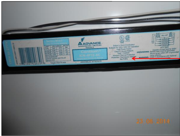
Photograph 48 Typical Advance Ballast, No Polychlorinated Biphenyls (PCBs)
