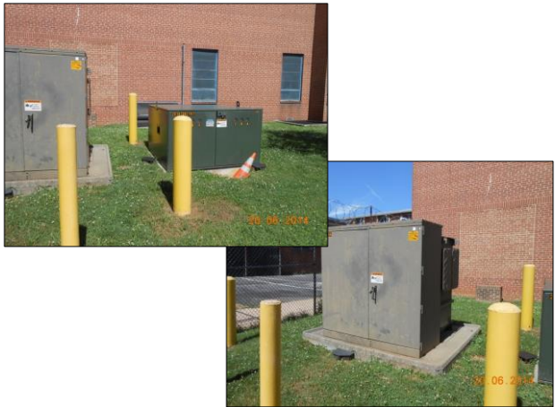
Photograph 53 Transformers, Exterior, Suspect for Polychlorinated Biphenyls (PCBs)
