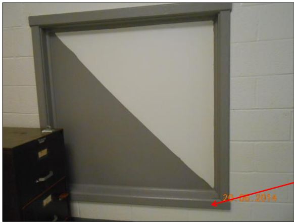
Photograph 43 Window Frame, Room 59, Lead Paint
