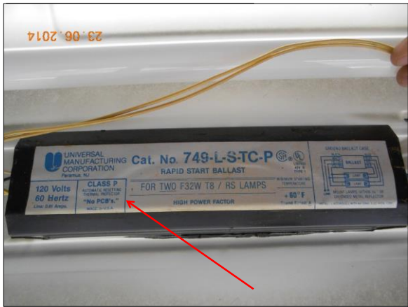
Photograph 49 Typical Universal Ballast, No Polychlorinated Biphenyls (PCBs)
