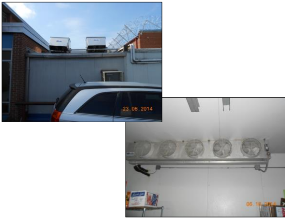
Photograph 56 Commercial Chiller Unit, Room 112 and Exterior, Ozone-Depleting Compounds (ODCs)
